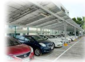
PV Module with Blocking Water Function
